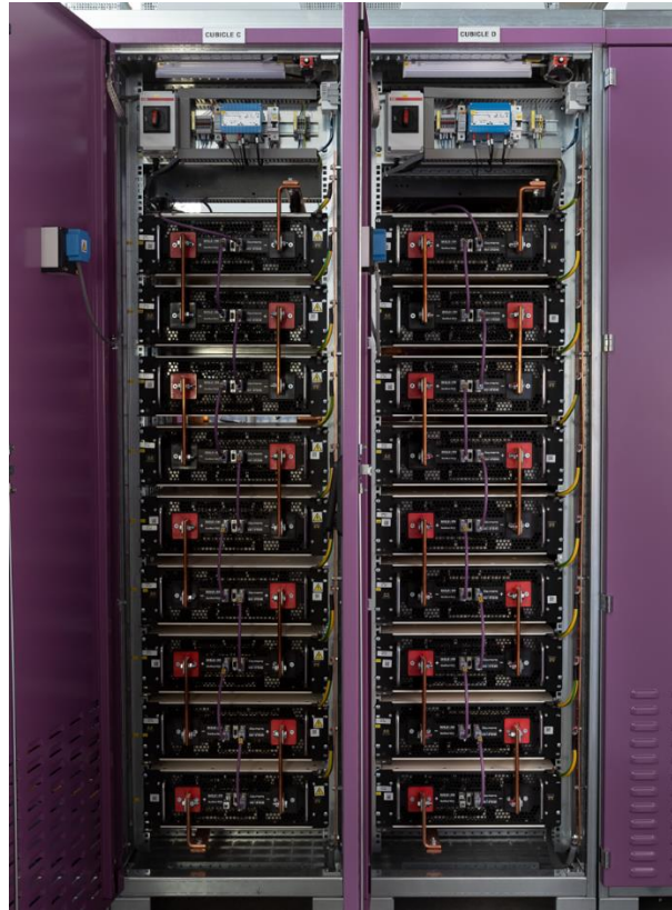
Figure 4 Supercapacitor bank made for Tokamak Energy
